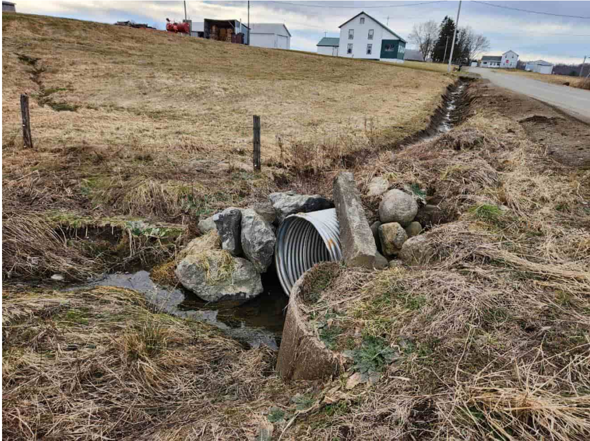
Photograph of existing culvert HH-3 configuration
